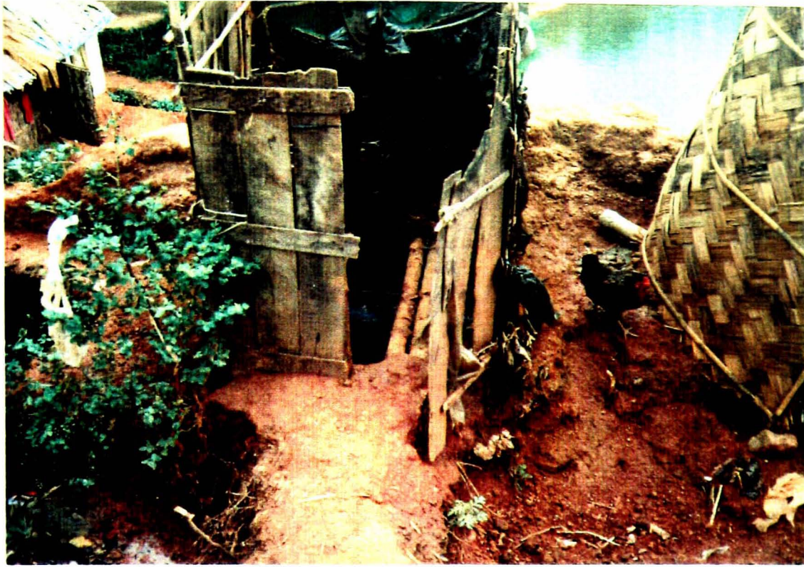
Plate 5. Hanging or kuccha latrine ( communal)
