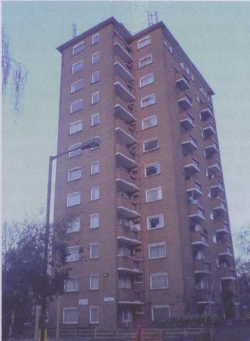
Figure 8 – Flick’s crack house
