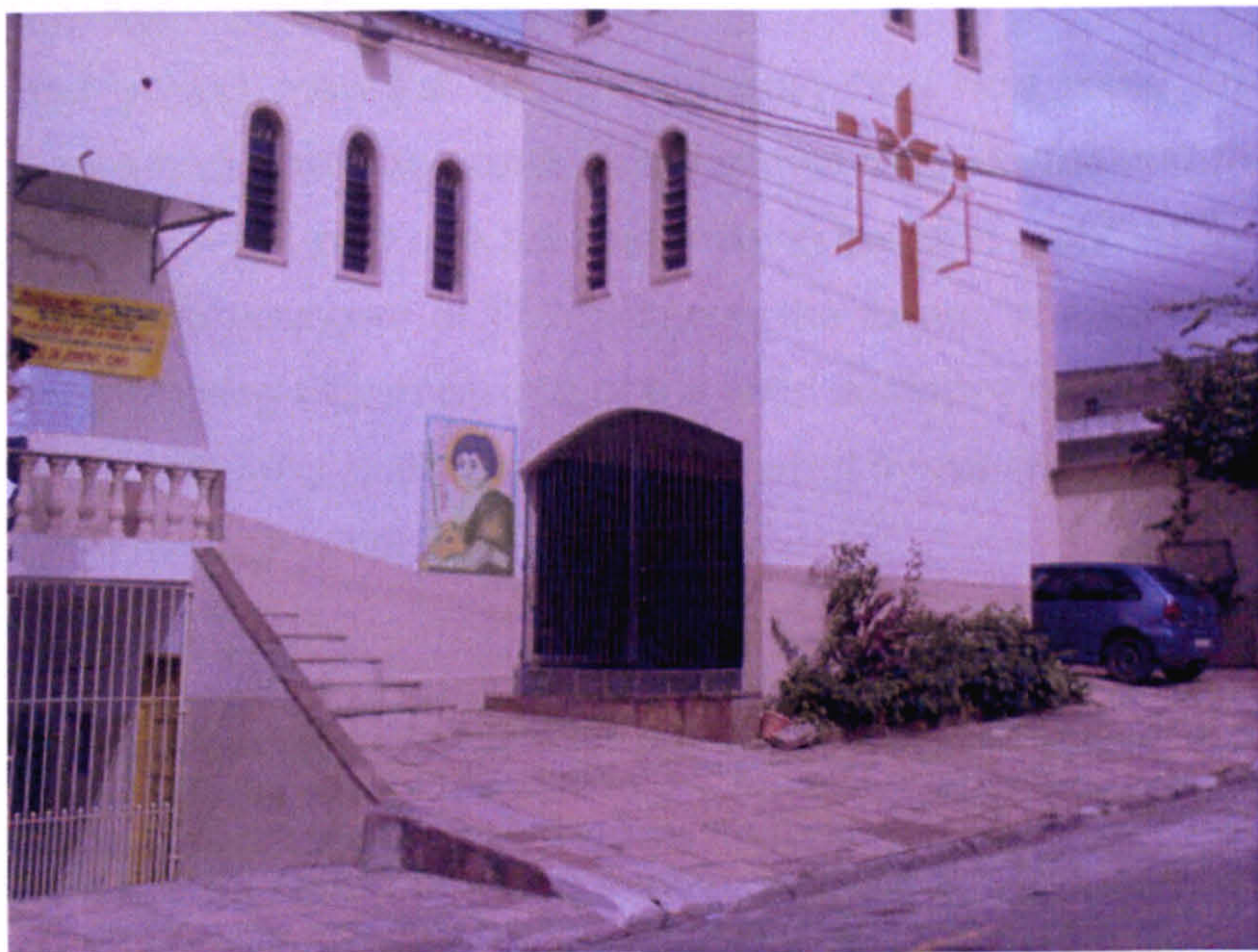
Figure 6 The RAC Building from the front
