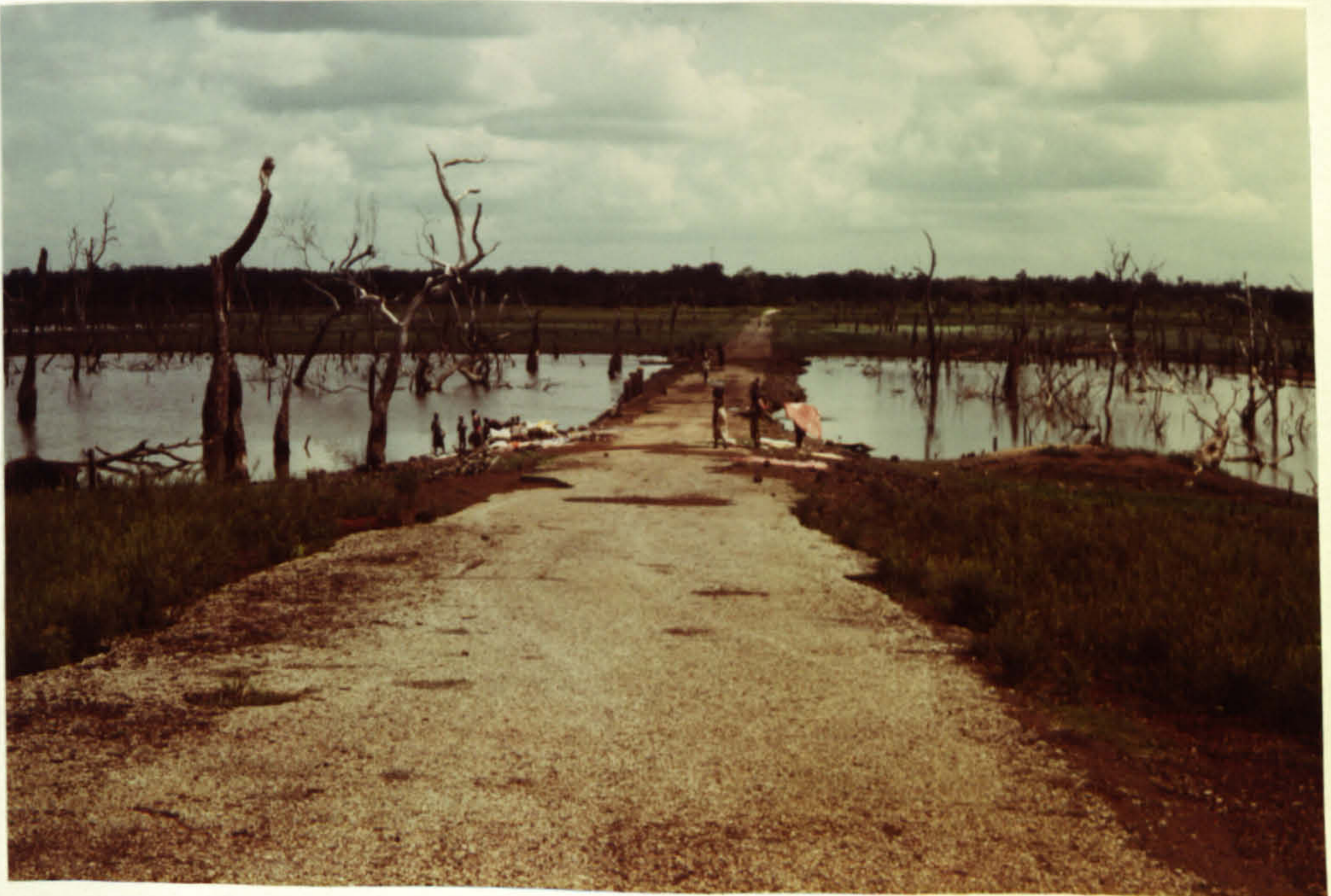
Plate 40. The main WCP at Prambo in June 1980.
