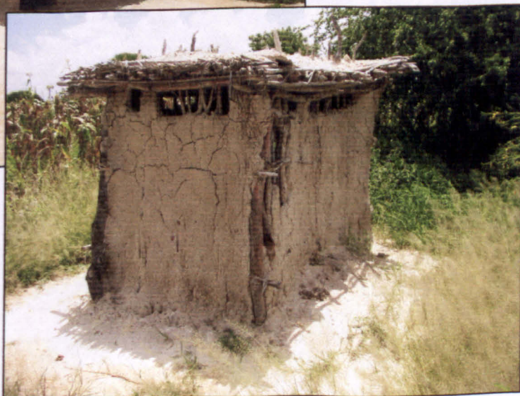
Photo 3.11 Chipanga "B" village: example 2 of roofed latrine
