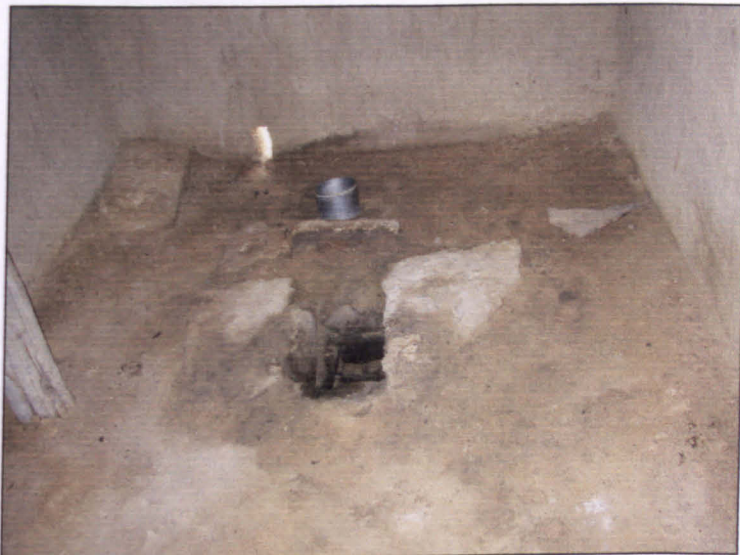
Photo 3.5 Lamaiti village: interior of cement-plastered latrine
