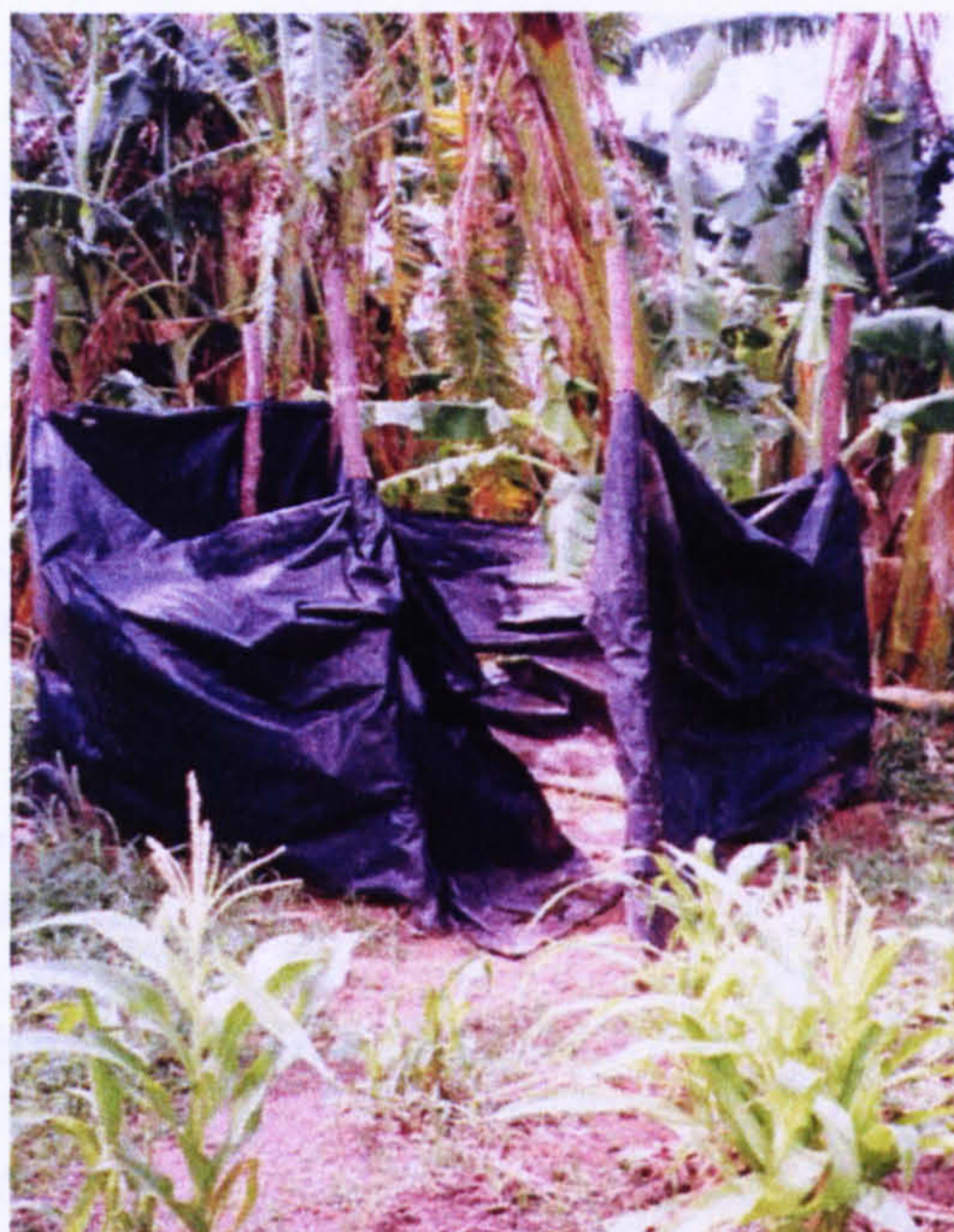
Figure 7-1: Typical latrine superstructure
