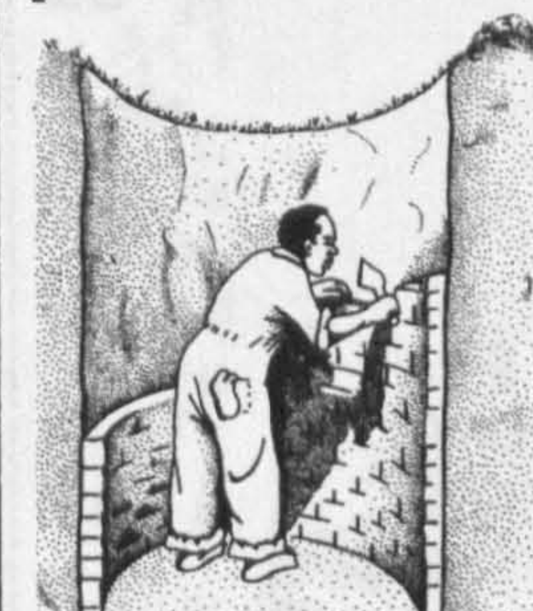
Lining the pit
