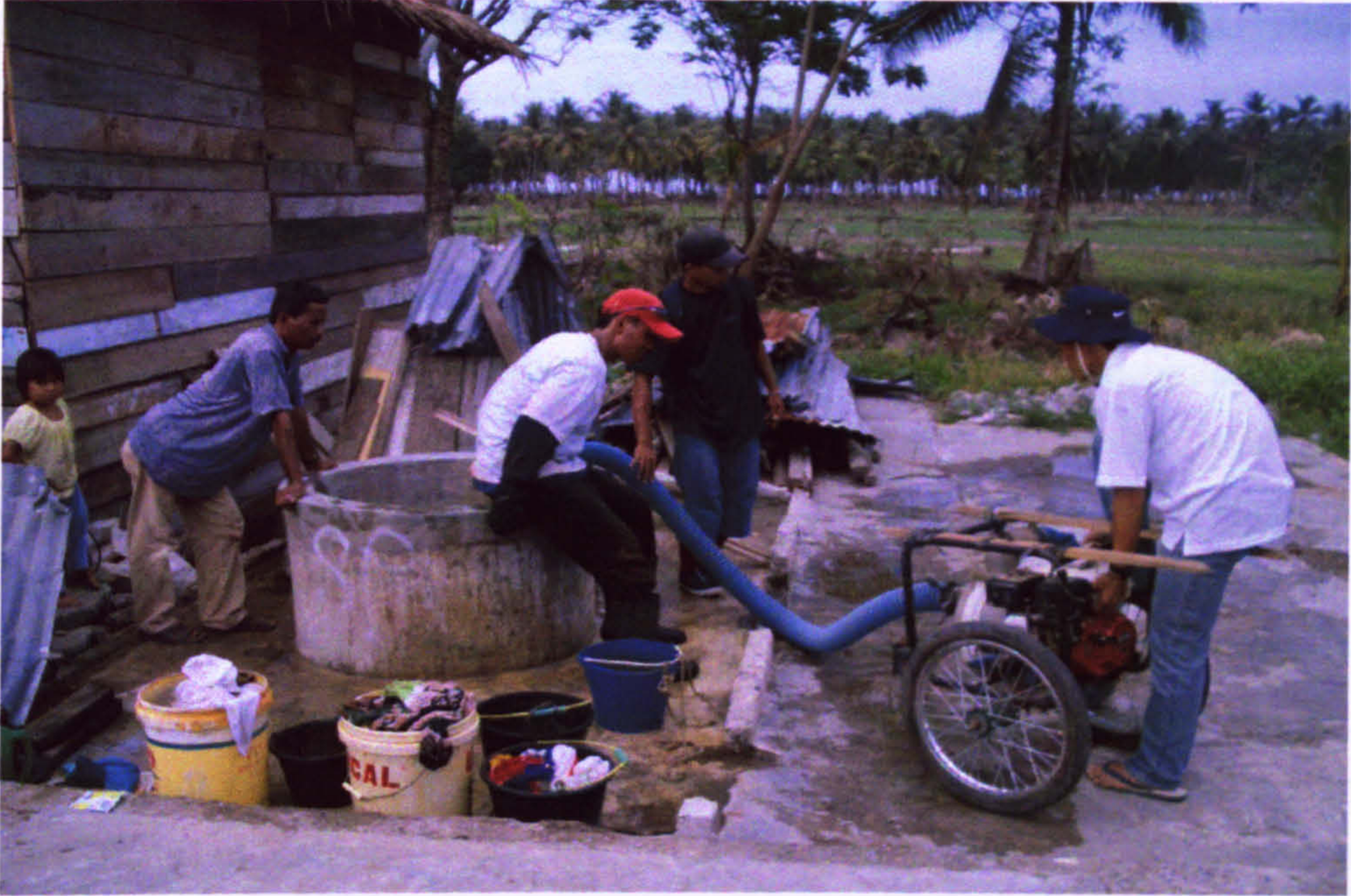
Figure 9.3.2d: Well refurbishing, Meulaboh, Indonesia
