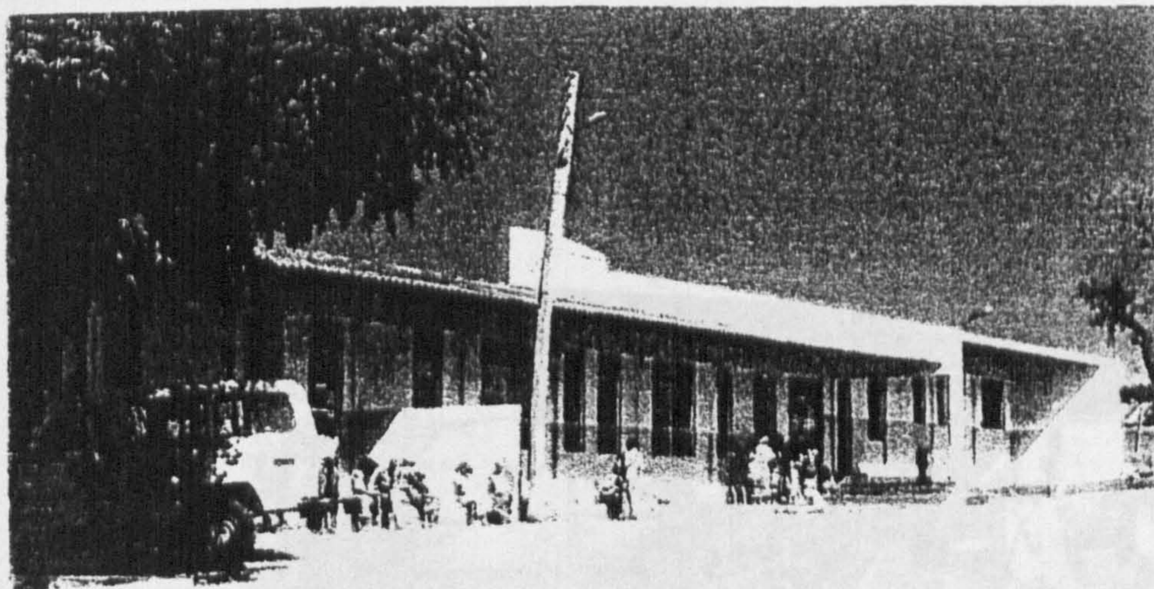
Picture 4.1: The Boane Health Centre
