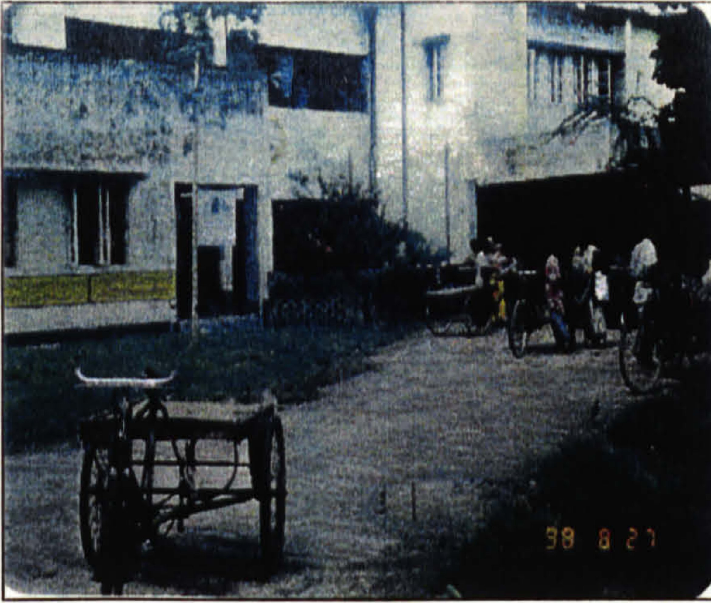
Photo 4.1 Front view of Keshabpur THC
