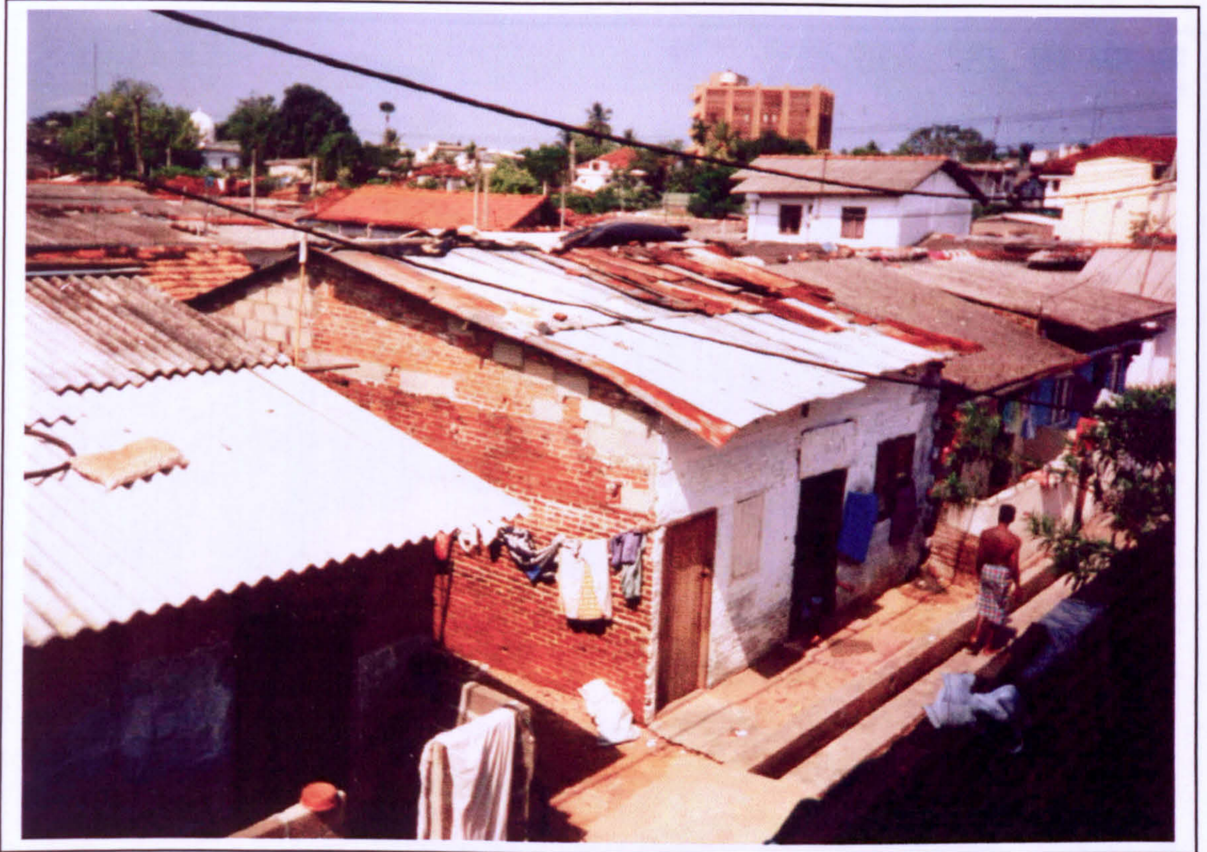
Photo 1: Improved infrastructure in Areas A, B and C: brick housing, drainage, sewers and electricity.
