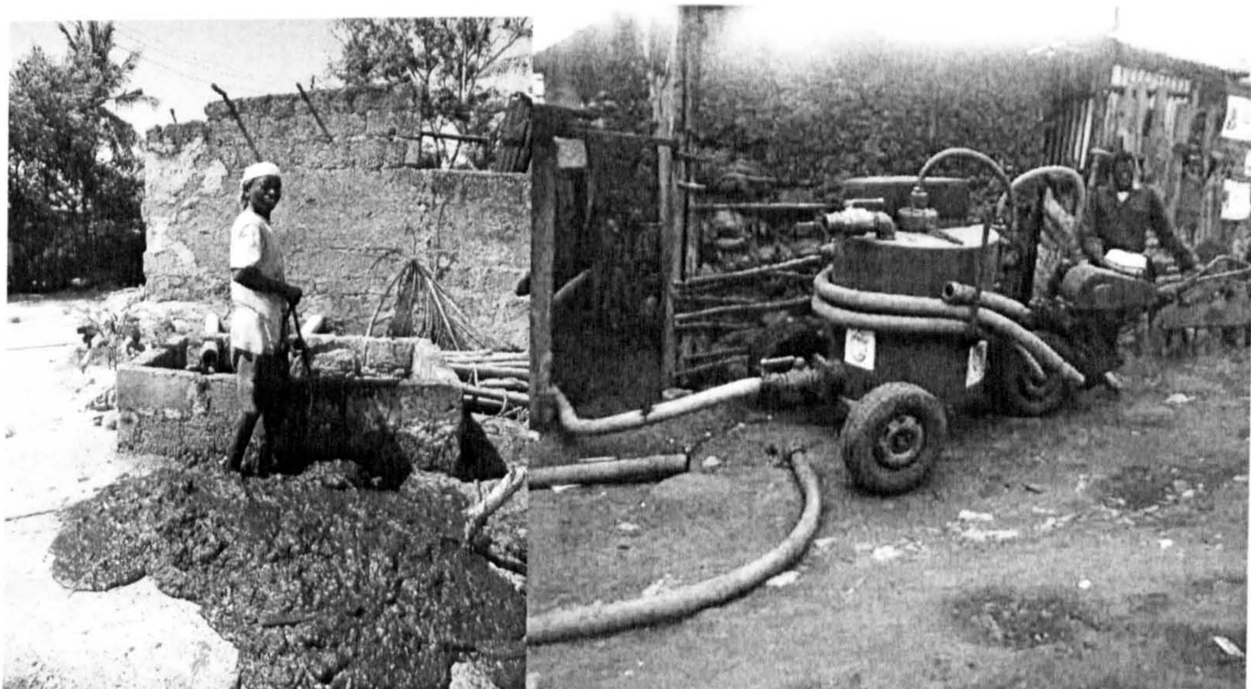
Figure 4.9: Manual and mechanical pit emptying methods for on-site sanitation
