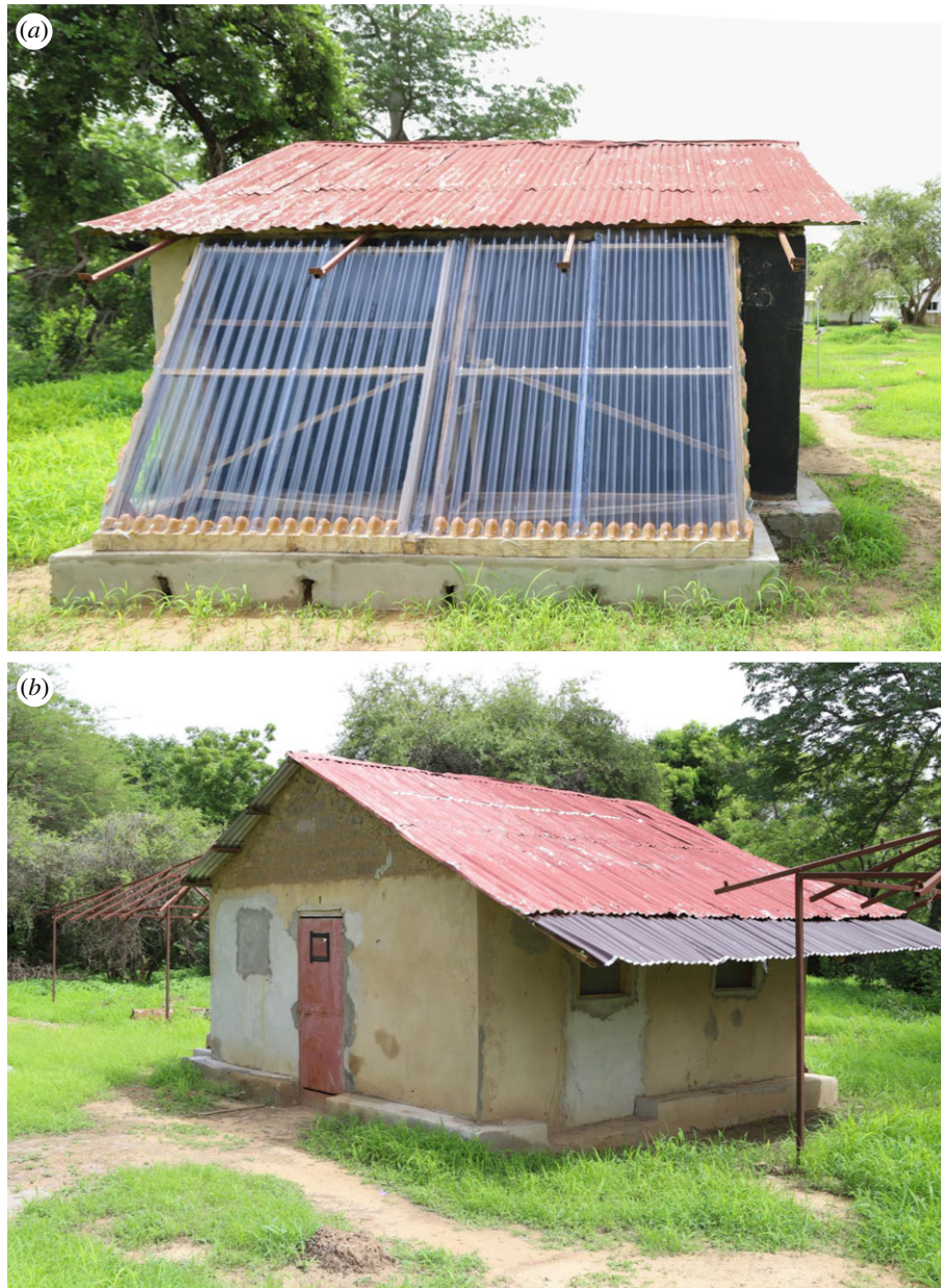
Figure 3. Experimental house with solar chimney on southeast facing wall (a) and extended roof on northwest elevation (b).
