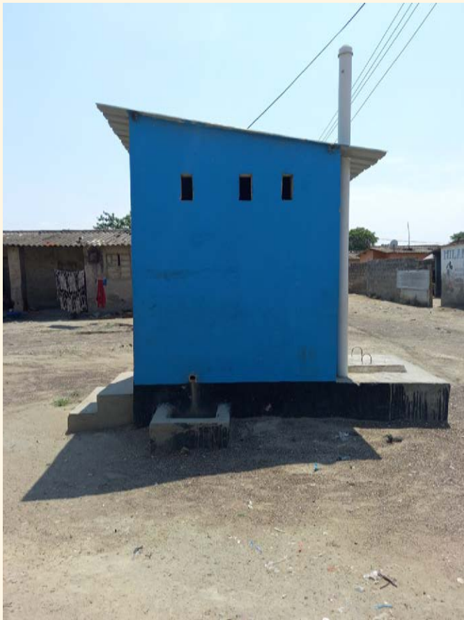
VIP dry Pit latrine - constructed under the Lusaka Sanitation program
