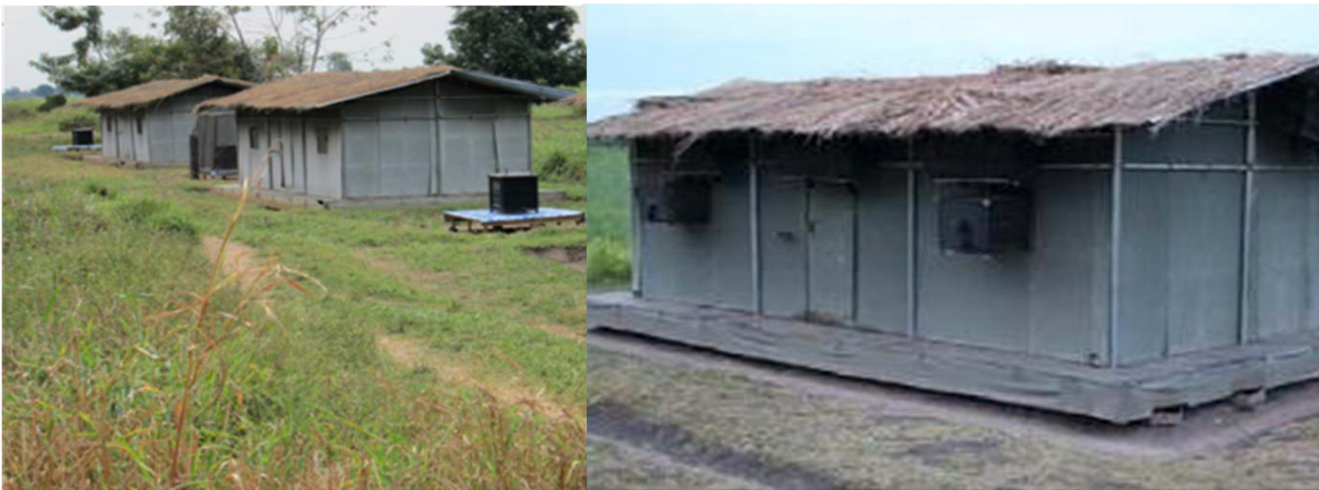
Figure 2. Ifakara experimental hut 27 . These are single-room model huts for entomological studies. They have eave spaces to allow mosquito entry and can be fitted with interception traps on these eaves and windows to collect mosquitoes as they exit from the hut.
