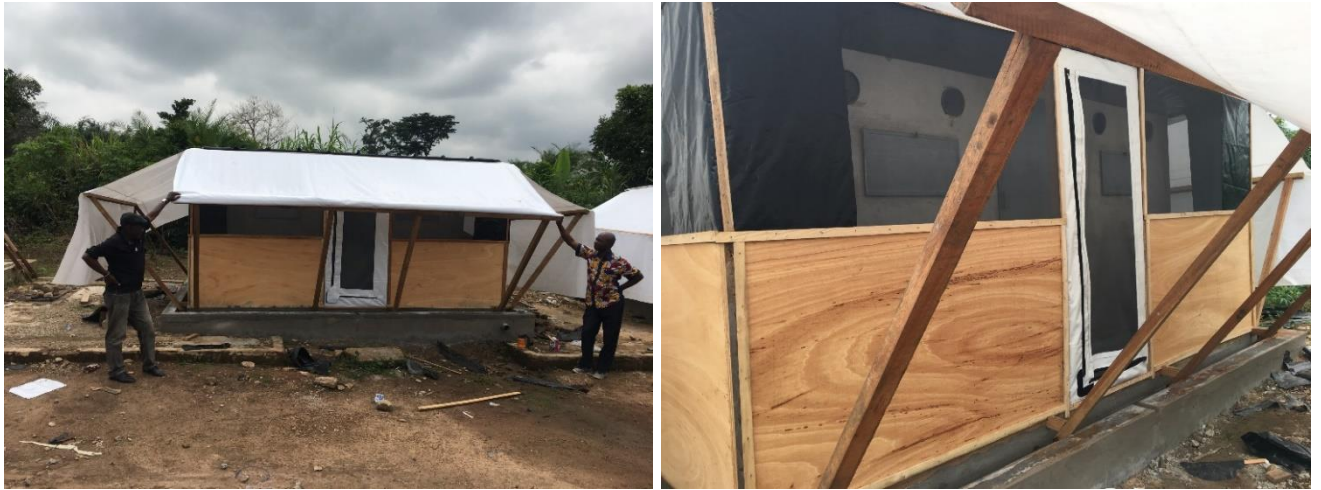
Fig. 7.1 Picture of the experimental hut fitted with EaveTubes
