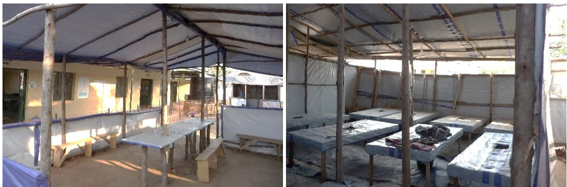
Figure 2-7 Cholera treatment centre of Uvira: communal areas for carers (left) and pre-admission observation area
