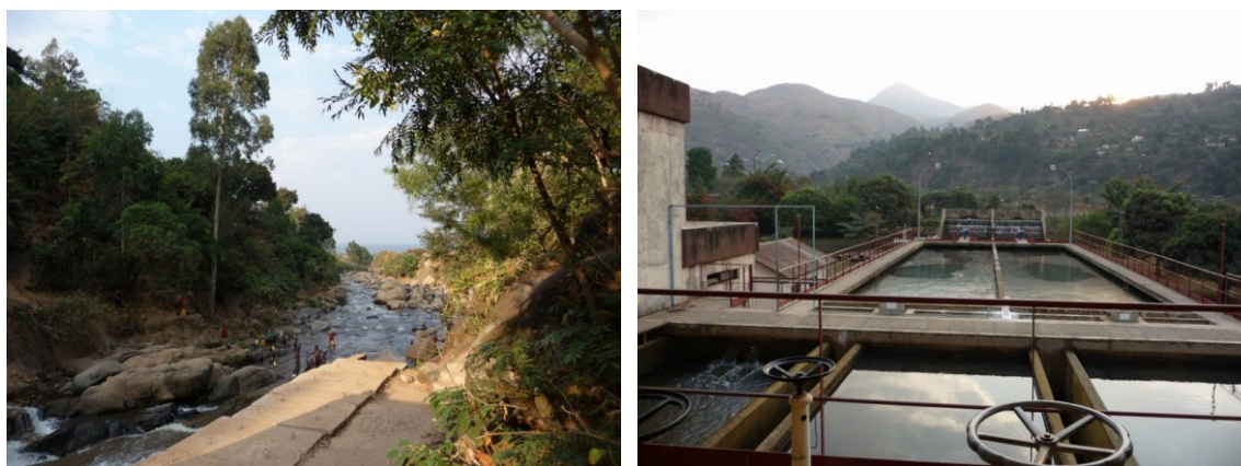
Figure 2-10 Water intake chamber on the river Mulongwe (left) and decantation reservoirs at the water treatment station (right)
