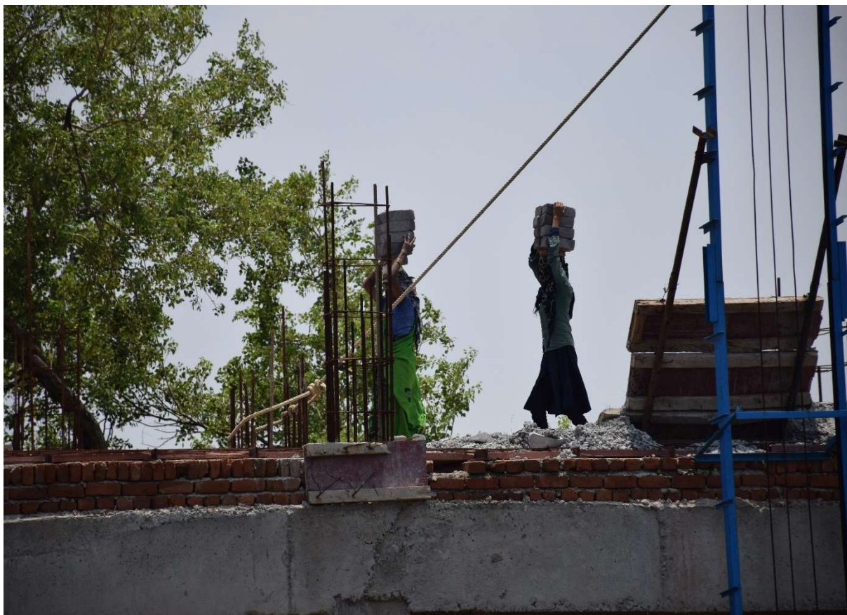
Photograph 1E: Female Construction Workers Carry Heavy Head Load
