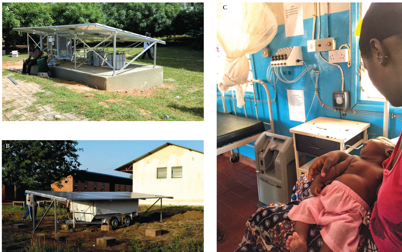
Figure 2. Solar-PS systems in the field. Panel A: Standard Solar-PS systems in situ in AFPRC Hospital, Farafenni, The Gambia. Panel B: Trailer Solar-PS system installed at Soma Health Centre, Soma, The Gambia. *Wheels were subsequently removed and fence erected to deter theft. Panel C: Trailer Solar-PS system supplying oxygen to a child in Soma Health Centre, Soma, The Gambia. *Photograph used with permission of caregiver.
