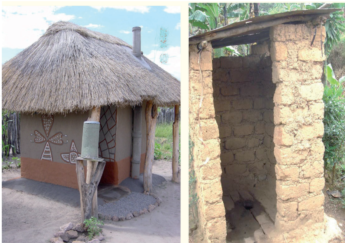
Figure 2. Left: Subsidized ventilated improved pit latrine (VIP) in a CHC home in Zimbabwe with lined pit, concrete slab and vent pipe - a fly trap which eliminates smell and a hand washing facility. Right: An unsubsidized traditional pit latrine in Rwanda, unlined and open pit, log floor giving open access for flies. Photographs courtesy of J. Waterkeyn.
