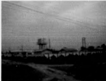
Legislators Quarters. Overhead Water Reservoir
