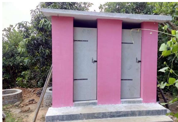
Figure 3.4 MANTRA-promoted sanitation and hygiene block. Improved, onsite toilet and enclosed, on-site bathing room infrastructure promoted via Gram Vikas' MANTRA programme. Photo: Gram Vikas via S. Thomas
