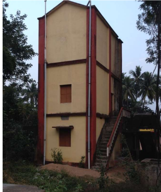
Figure 3.5 MANTRA village water tower, tank. The village water tower constructed with support from Gram Vikas houses a tank on the top floor, and a village meeting room on the bottom floor. Photo: M. Delea
