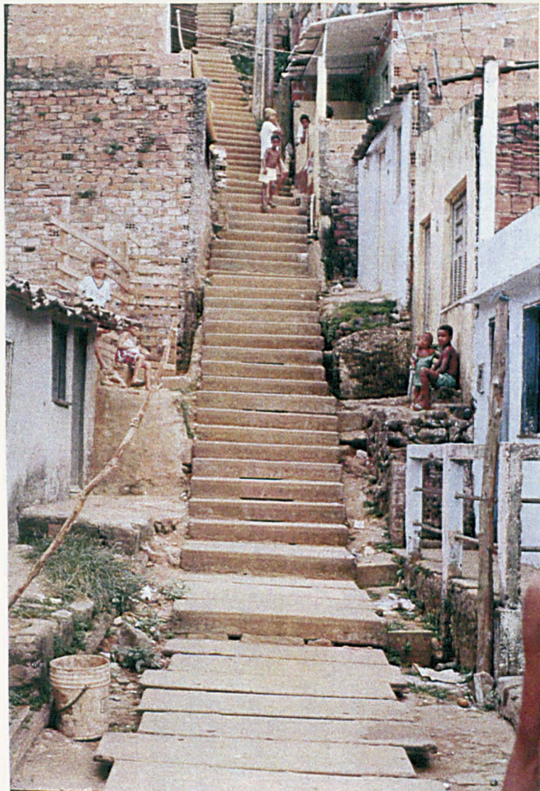
Photo 2. Stairways and ramps drainage system in the Antônio Balbino neighbourhood
