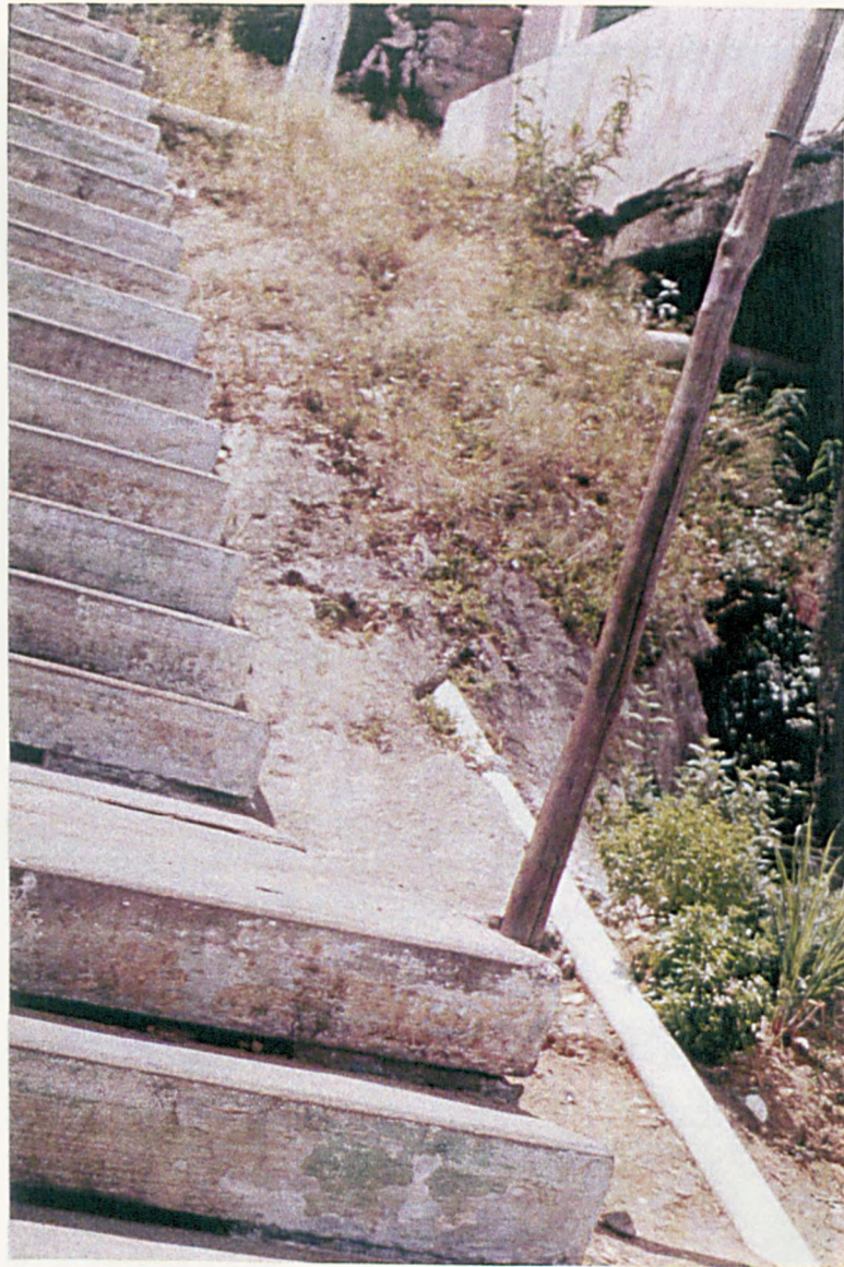
Photo 1. Shallow sewerage and stairways drainage system in Boa Vista de S. Caetano neighbourhood
