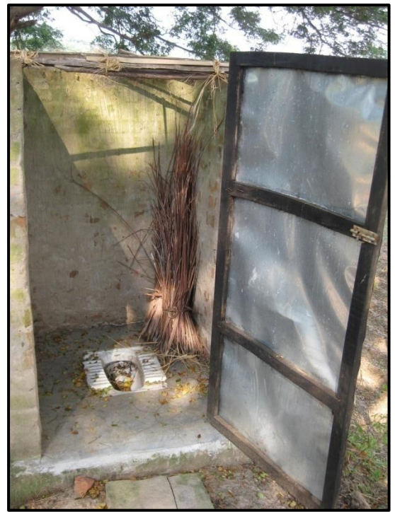
Figure 6. An unused completed latrine in Sankhatira village
