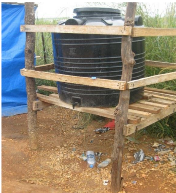
Figure 6: Handwashing station at entrance of UN House
