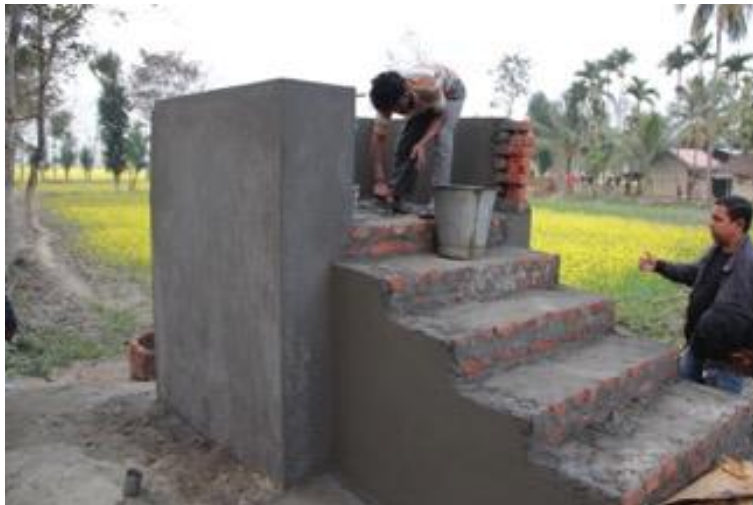
Figure 1: Raised concrete platform with steps for water source by Action Aid
