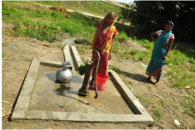
Figure 2: Concrete platforms for handpumps provided by Oxfam
