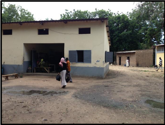
Figure 7.1 Two health facility exteriors to highlight impact of Results-based Financing pilot
