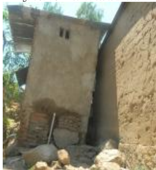
Figure 5.2: UDT built close to a house
