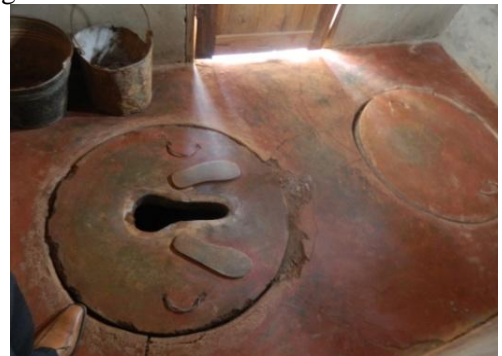
Figure 3. 2: Interior view of fossa alterna toilet
