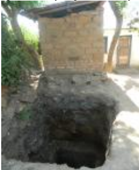
Figure 5.1: New pit dug on old latrine spot
