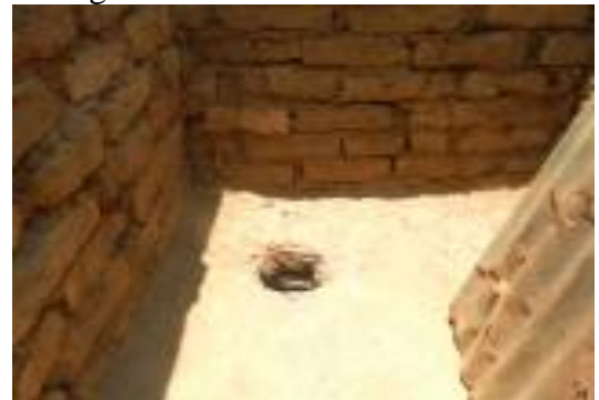
Figure 3. 5: Pit latrine - mud floor
