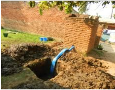
Figure 6. 1: Pit latrine being emptied
