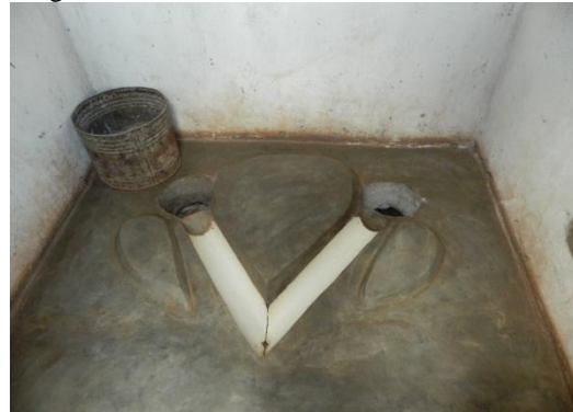
Figure 7. 3: UDT with bucket for ash and soil
