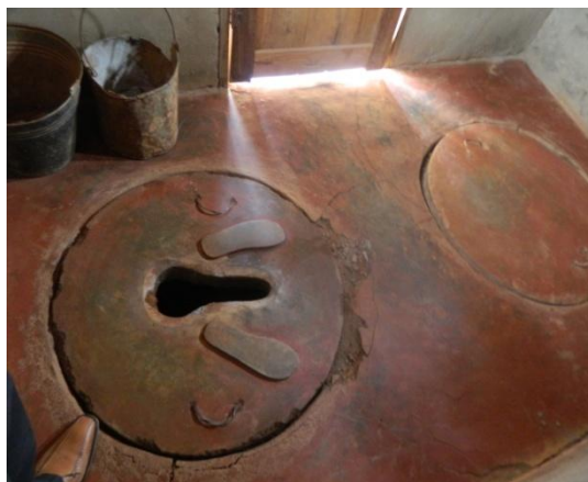
Figure 1. 3: Twin pit fossa alterna with one hole in use and another one closed.
