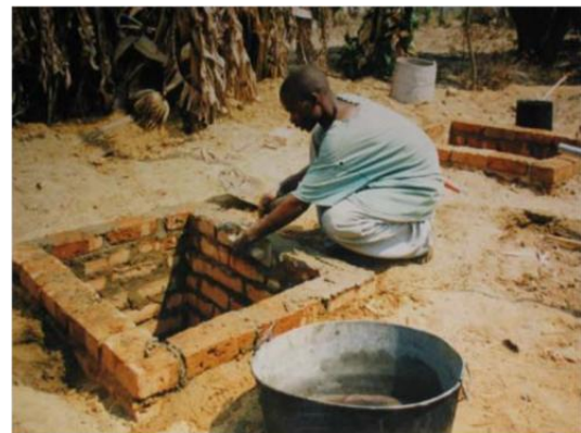
Figure 5.4: Lining pit with bricks (lined pit latrine)
