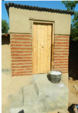
Figure 7. 1: UDT front view
