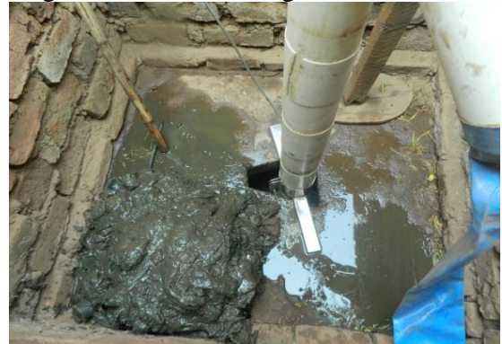
Figure 1.2: Faecal sludge on latrine floor
