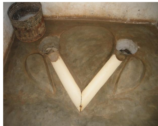
Figure 1. 4: Urine diverting toilet (UDT), with two holes that are used alternately.
