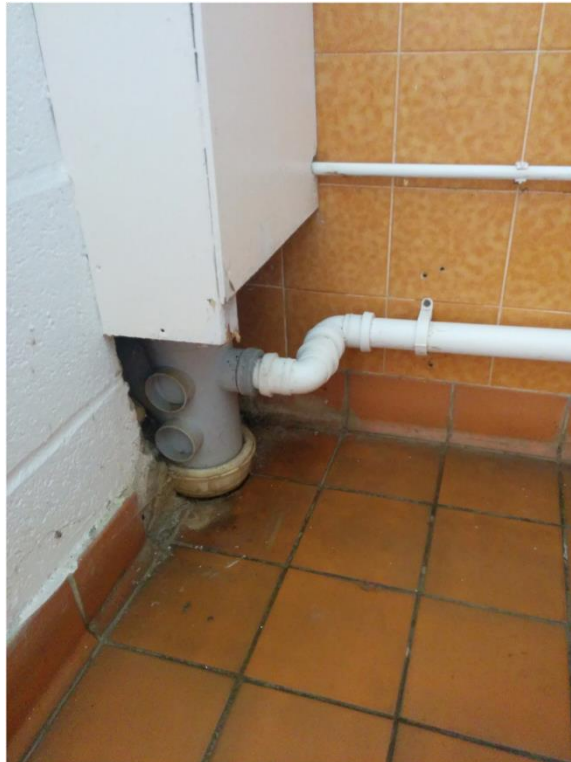
Figure 5.1: Photograph showing the primary collection area of resting mosquitoes in the toilet block at Elmley. Blood-fed Anopheles maculipennis s.l. mosquitoes were found resting directly on the walls and on or under the exposed wooden covering to the pipework.
