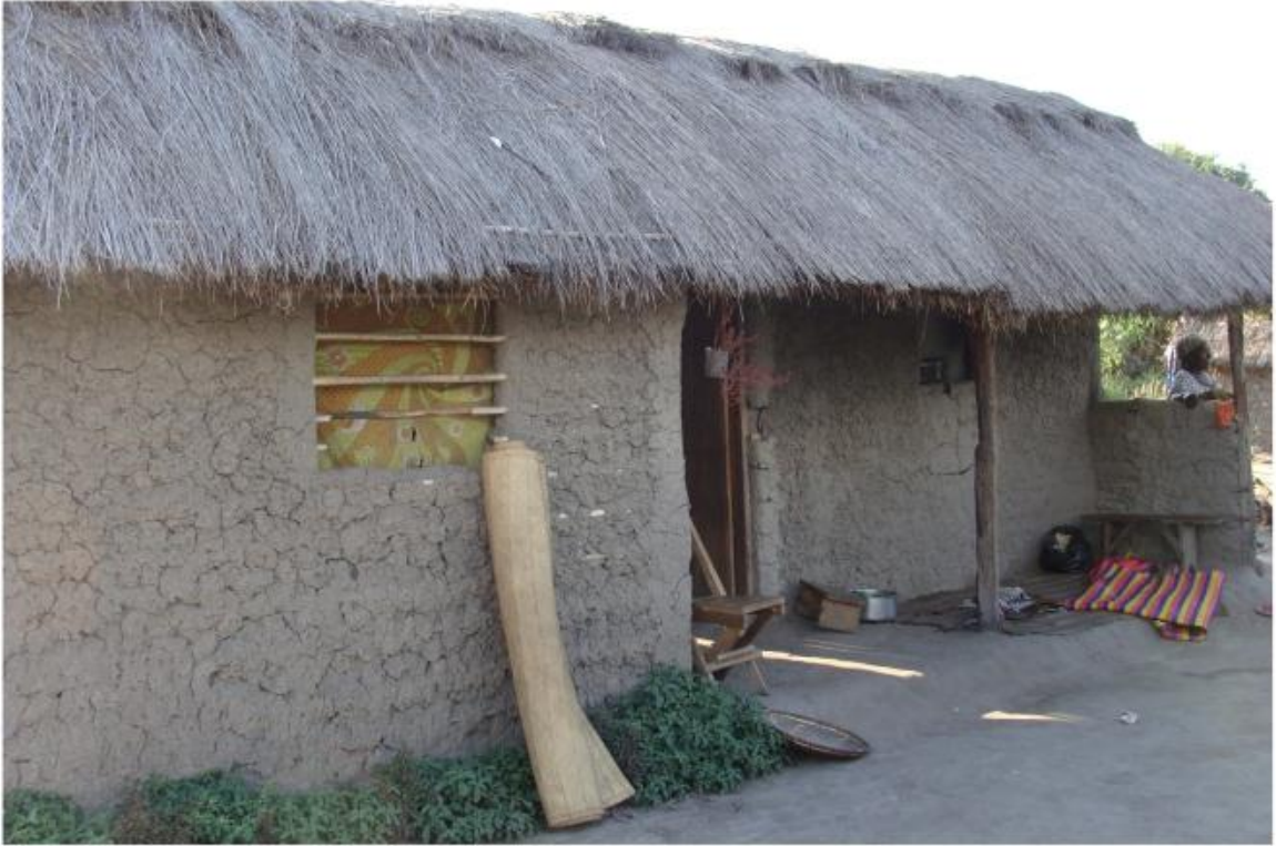
Figure 3.1. A local house. The local houses are made of mud walls and thatched roofs. They have one door and two windows and open eaves (open spaces between the roof and the wall).
