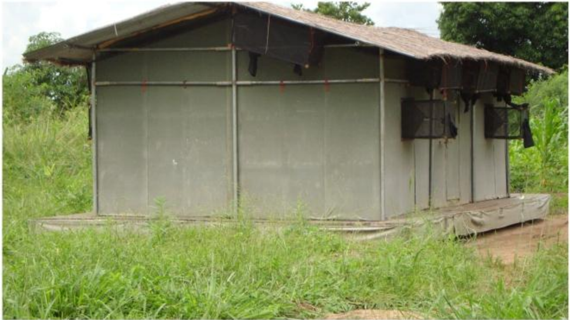
Figure 3.2. A wooden experimental hut. The experimental huts were designed to represent local housing in southern Tanzania. An experimental hut had a corrugated roof and covered with grass thatch on the top, to simulate the temperature of local houses with thatched roofing. The outer walls were constructed from wooden planks or canvas. The inner walls were made of removable panels coated with mud. They had one door and two functional windows with open eaves (open spaces between the roof and the walls).
