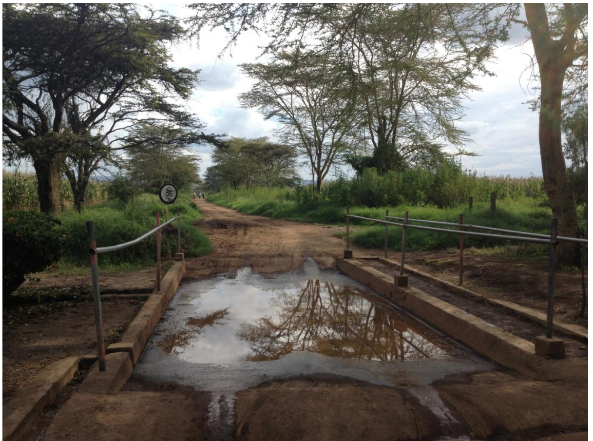
Figure 11.4. Photograph of wheel bath present on Farm 1/SAT2. The bath is not in use with only rainwater being present.
