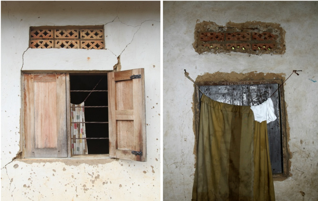
Fig 1. External (left) and internal (right) view of unscreened airbricks.
