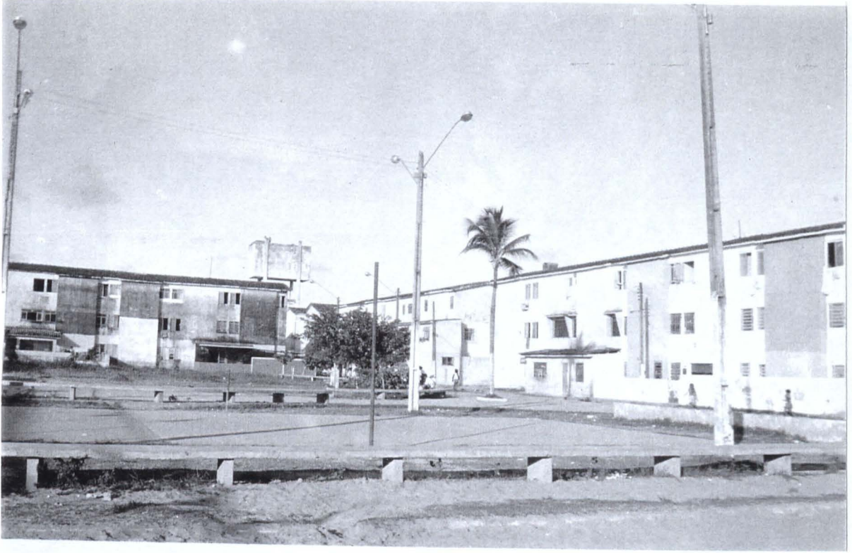
FIGURE 3.4 - LOW-INCOME APARTMENT BUILDINGS IN JARDIM BRASIL
