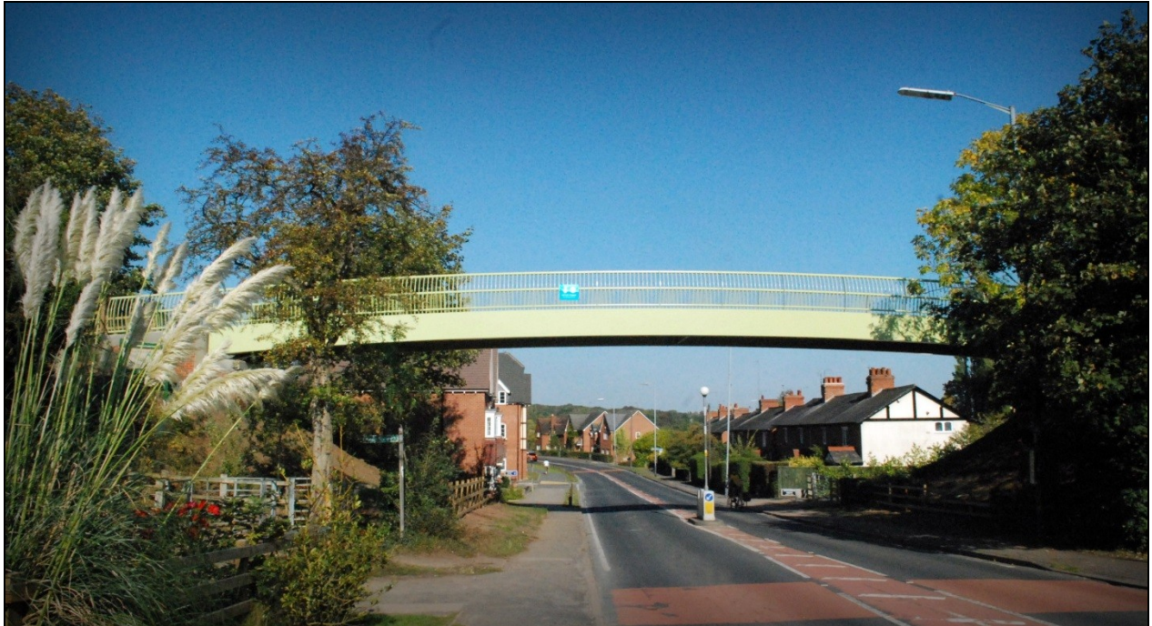
Figure 2: Illustration of the ‘core’ (flagship) element of the Kenilworth Connect2 scheme, a walking and cycling bridge
